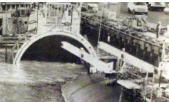
The first ever waterborne removal of a submarine sonar dome at Mare Island Naval Shipyard in June 1994 from the Baton Rouge (SSN-689). All pictures appeared in the 10 June 1994 issue of the shipyard's newspaper the "Grapevine". The first of four photos appears (top left). Divers begin the process of removing the dome cone. (top right) Workers begin the process of separating the dome. (bottom left) The dome is separated and waters fill the interior section of the Baton Rouge (SSN-689). (bottom right) The dome is completely removed from the Baton Rouge (SSN-689) and is raised from the water.
