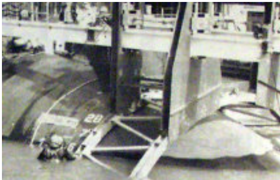
The first ever waterborne removal of a submarine sonar dome at Mare Island Naval Shipyard in June 1994 from the Baton Rouge (SSN-689). All pictures appeared in the 10 June 1994 issue of the shipyard's newspaper the "Grapevine". The first of four photos appears (top left). Divers begin the process of removing the dome cone. (top right) Workers begin the process of separating the dome. (bottom left) The dome is separated and waters fill the interior section of the Baton Rouge (SSN-689). (bottom right) The dome is completely removed from the Baton Rouge (SSN-689) and is raised from the water.
