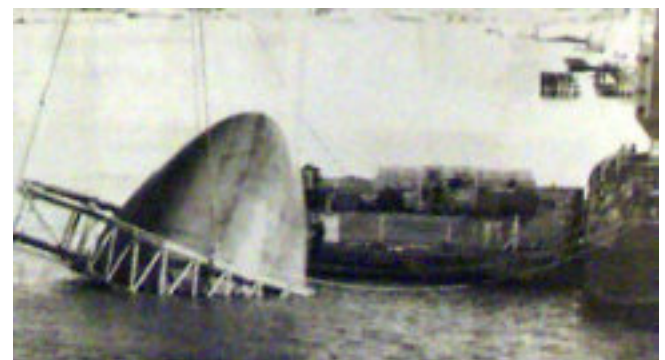
The first ever waterborne removal of a submarine sonar dome at Mare Island Naval Shipyard in June 1994 from the Baton Rouge (SSN-689). All pictures appeared in the 10 June 1994 issue of the shipyard's newspaper the "Grapevine". The first of four photos appears (top left). Divers begin the process of removing the dome cone. (top right) Workers begin the process of separating the dome. (bottom left) The dome is separated and waters fill the interior section of the Baton Rouge (SSN-689). (bottom right) The dome is completely removed from the Baton Rouge (SSN-689) and is raised from the water.
