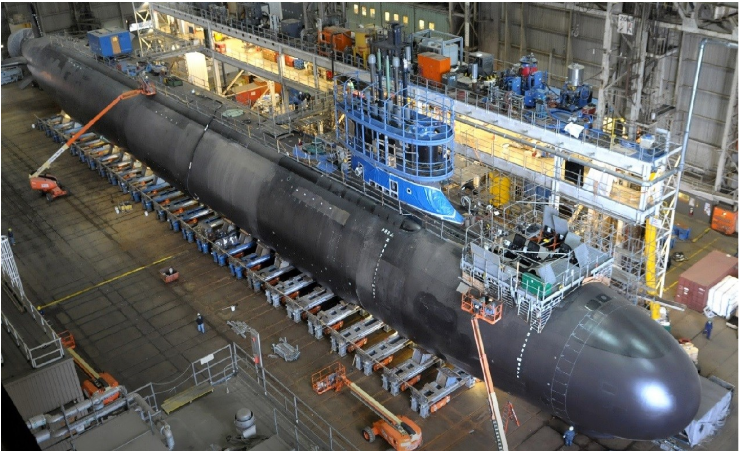
US Navy Virginia-class Submarine Under Construction.
