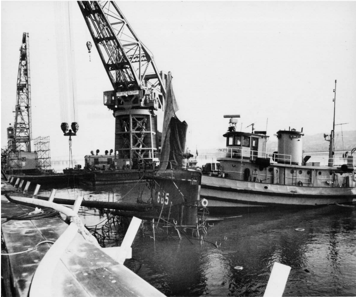
The Guitarro (SSN-665) is on the bottom of the Napa River after her accidental sinking at Mare Island on 15 May 1969. (Note: The reactor had not been installed). Other vessels in the picture are from left to right; unknown YD , YD-33 (150 Ton Crane), and Satanta (YTM-270). Satanta is preventing the Guitarro from capsizing
